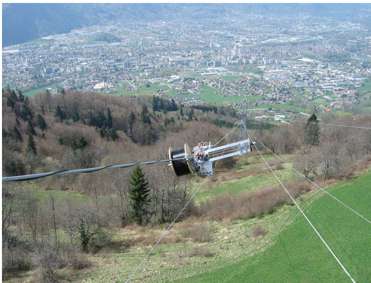
Figure 2 – Optic fibre cable installation AFL SkyWrap ( www.aflglobal.com )
