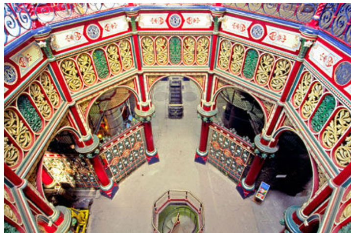
Pic: Crossness Engines as it stands today
